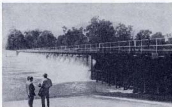
FIGURE 6. Dethridge weir in operation.
