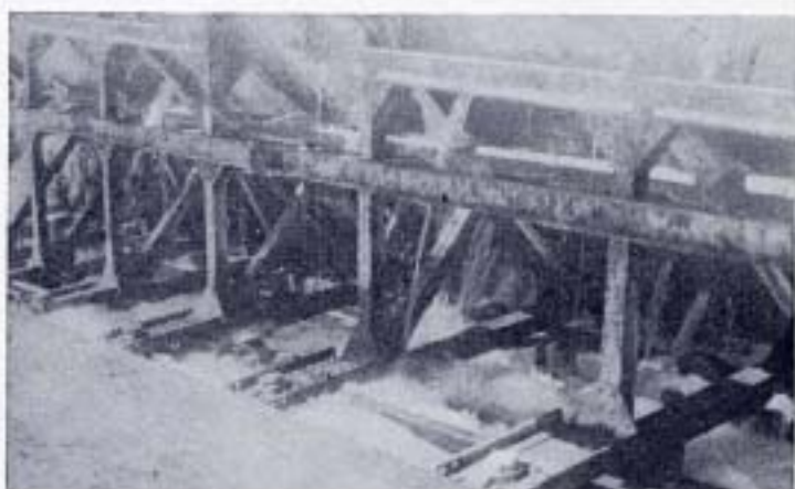
FIGURE 5. Close up of frames.
